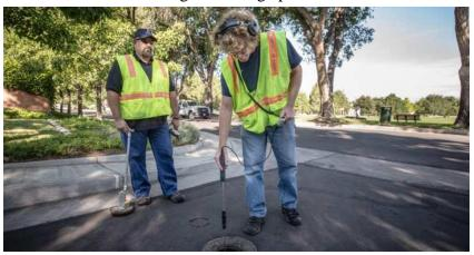
Detection of leakage by sounding rod method
