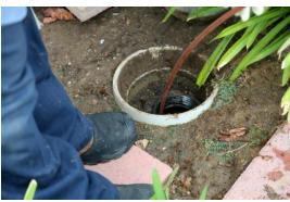
The sewers are tested by plugging the upper end with a provision for an air outlet pipe with stop cock. The water is filled through a funnel connected at the lower end provided with a plug. Afterwards the air is expelled out, stop cock is closed and the water level in the funnel is raised to 2.5 m above the invert at the upper end. The water level in the funnel is noted after 30 minutes and the quantity of water required to restore the original water level in the funnel is determined.
