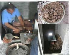
The teacher/ instructor is required to demonstrate to the students how to calculate the materials required for fixing Indian type water closet and installation of the same observing all health & safety requirements, policies and procedure of the authority. The students have to perform the same.
